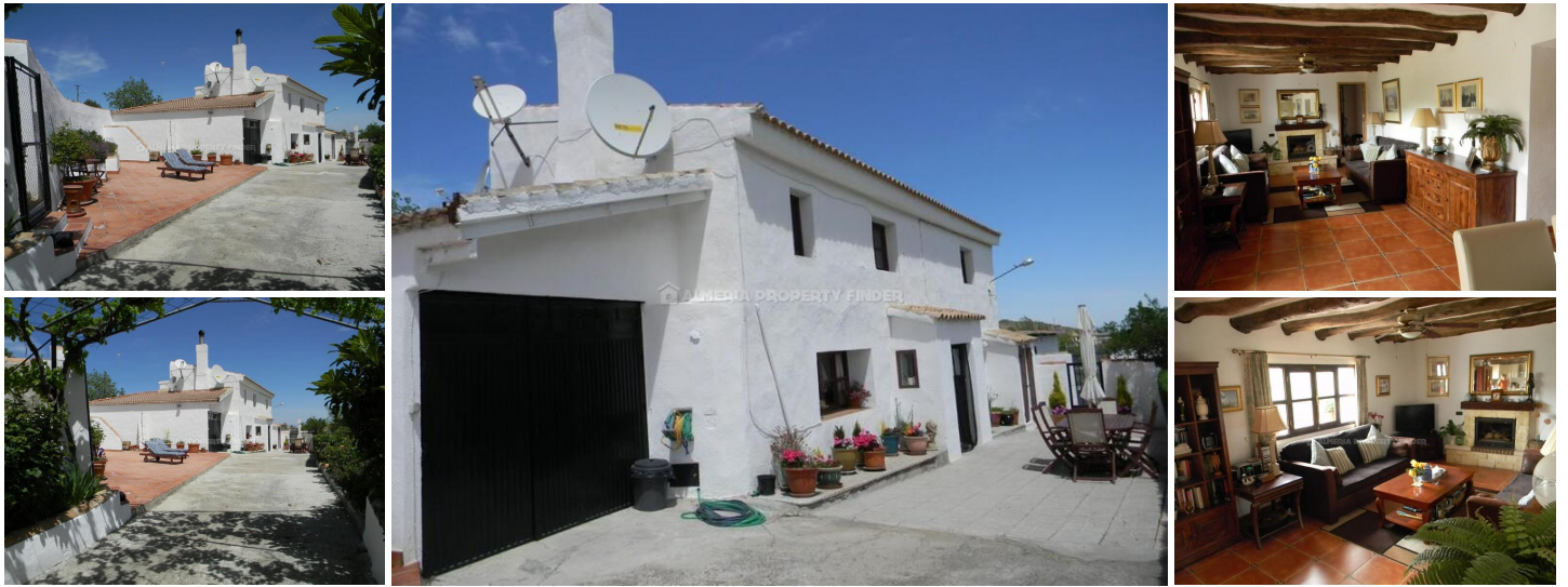
Cortijo Delauna - A country house in the Caniles area. (Renovated)
