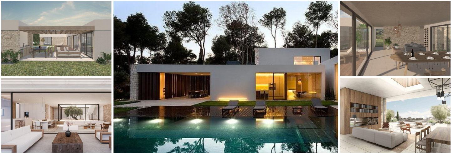
NEW BUILD VILLA IN YECLA, MURCIA
