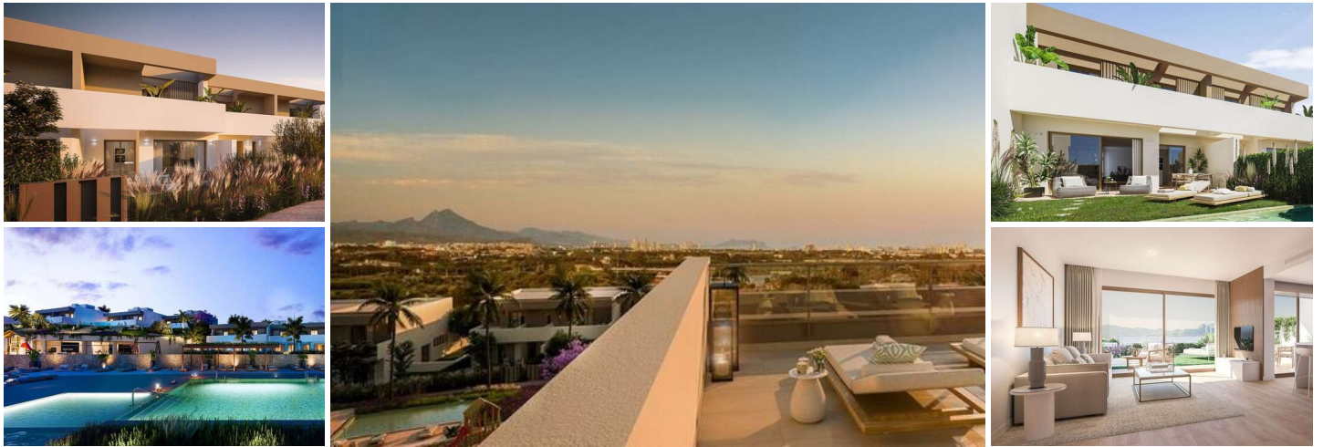
NEW BUILT CHALETS IN VISTAHERMOSA (ALICANTE)
