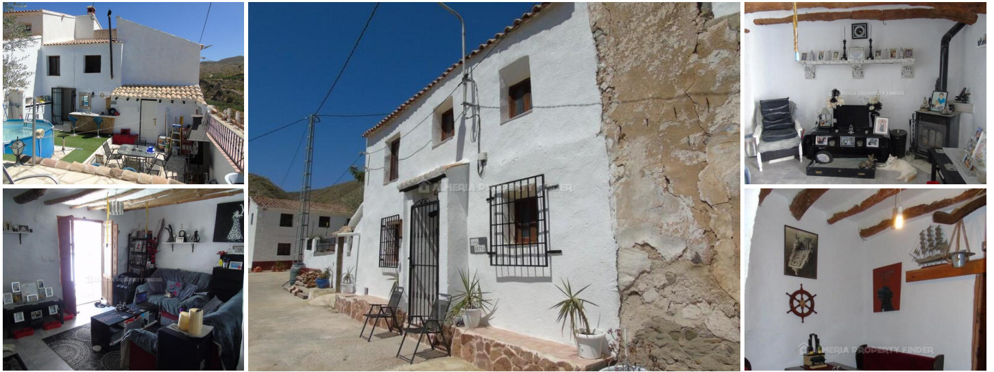
Cortijo Dante - A country house in the Arboleas area. (Renovated)
