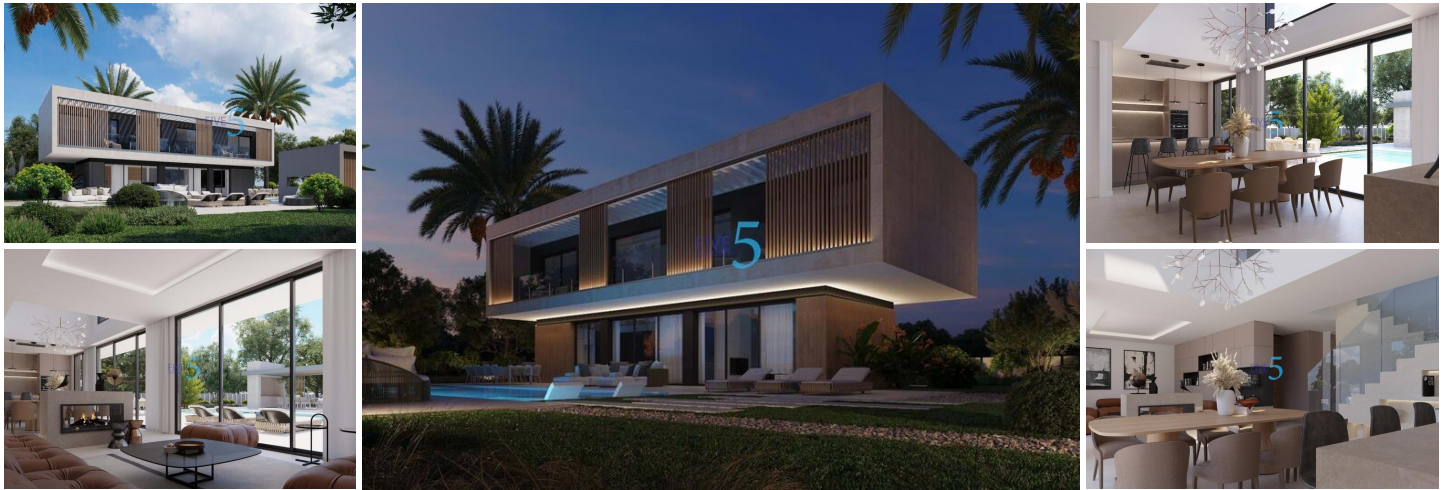
NEW BUILD VILLA IN JAVEA
