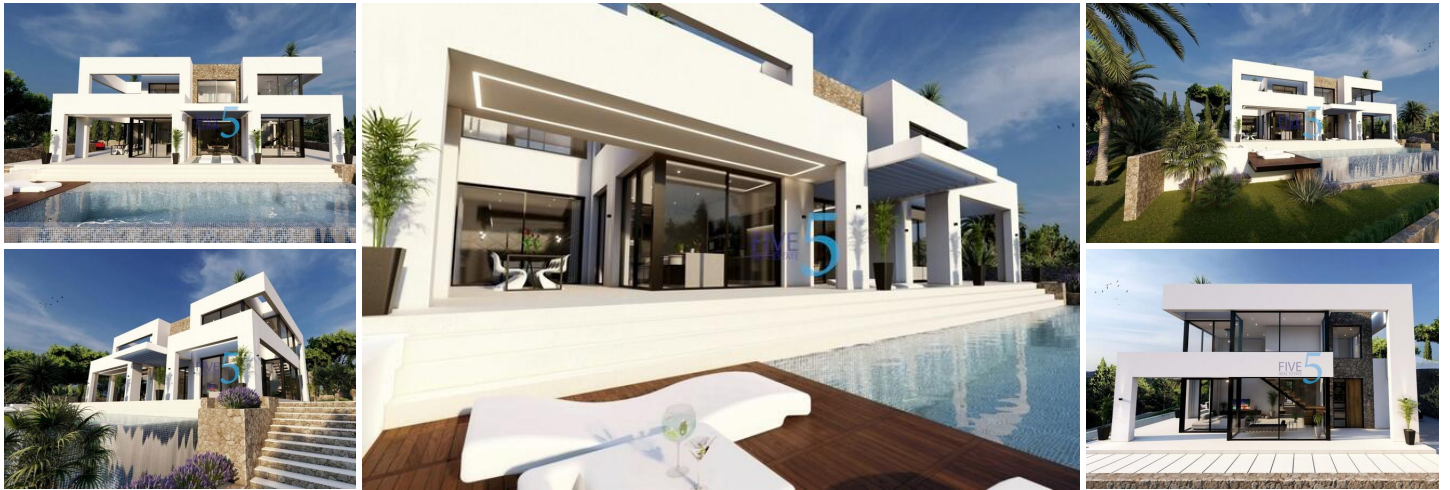
NEW BUILD VILLA IN BENNISA
