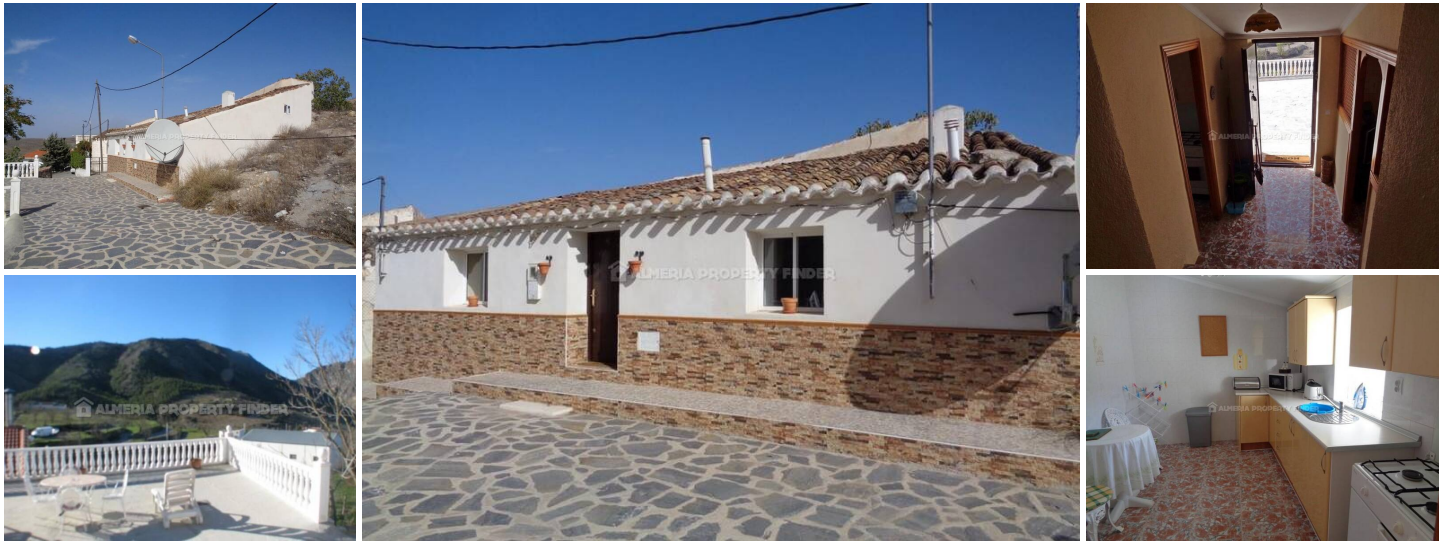
Casa Marie Dos - A village house in the Oria area. (Renovated)
