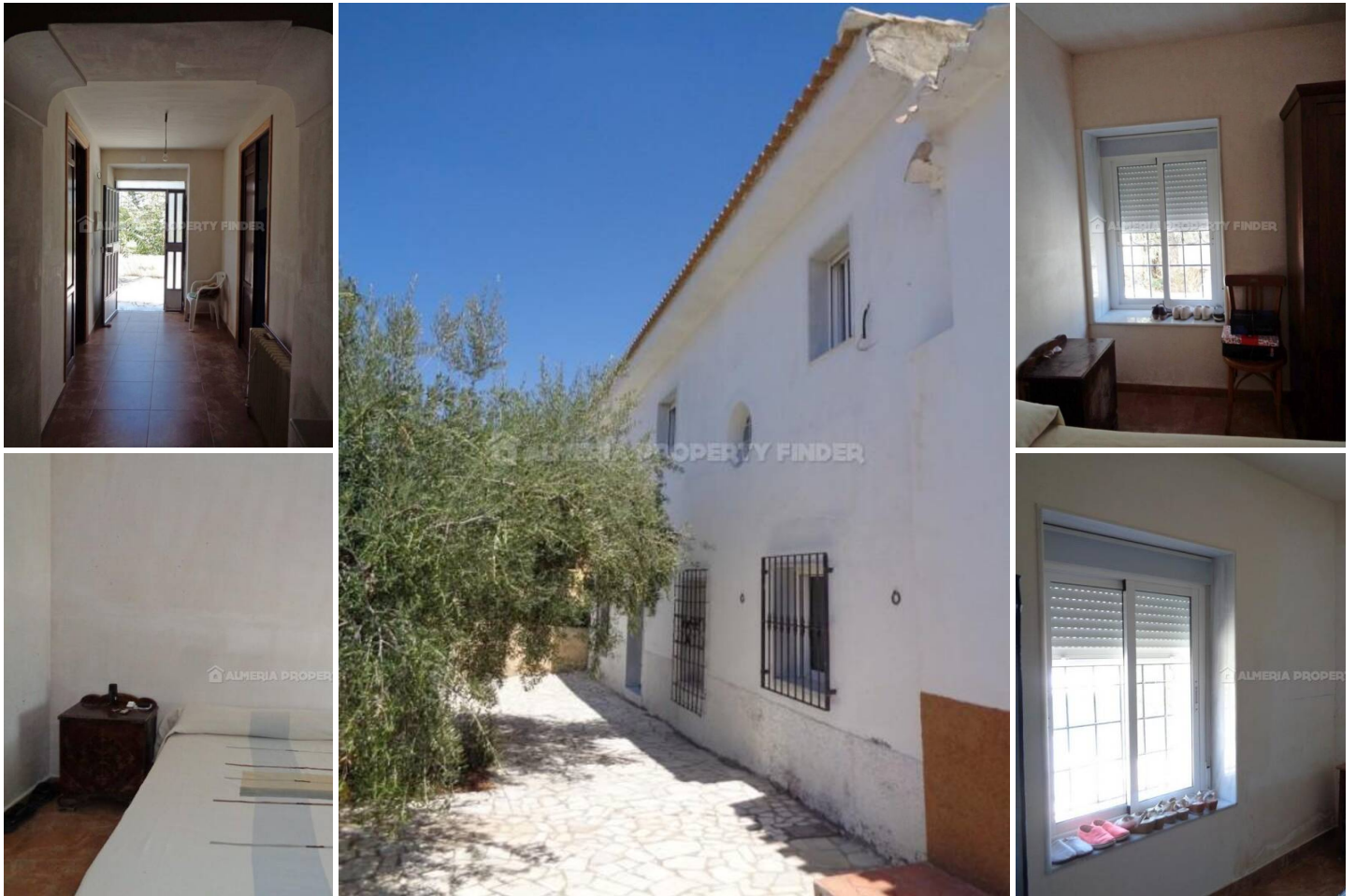
Cortijo Marques - A country house in the Albox area. (Renovated)
