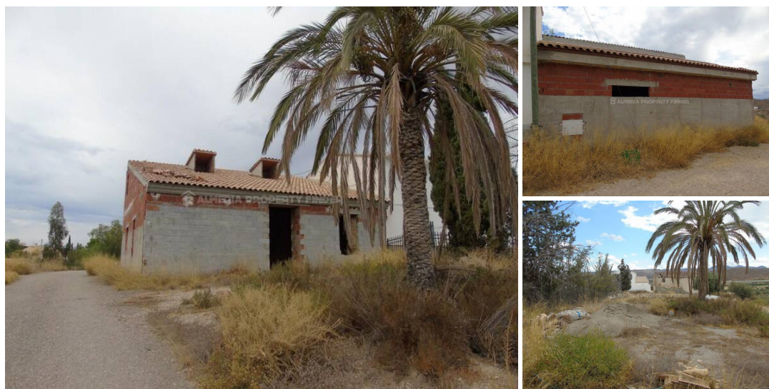
Casa Canico - A country house in the Albox area. (Under Construction)
