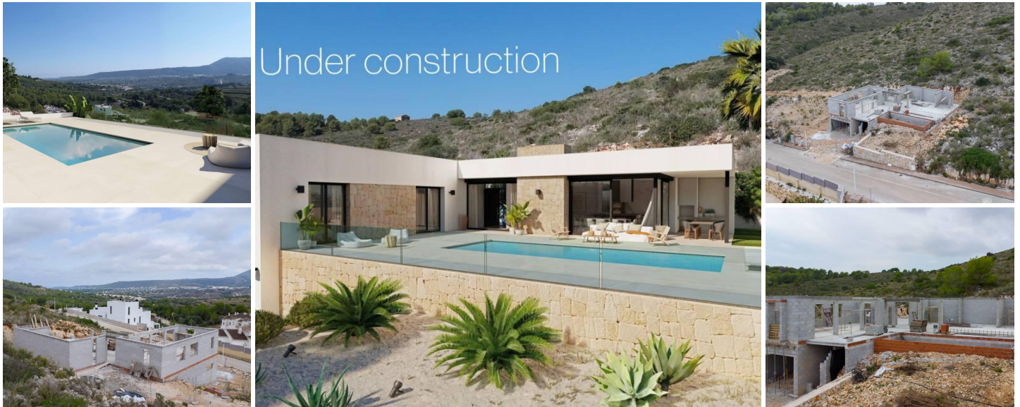
Modern new-build villa under construction for sale in Racó de Nadal, Benitachell
