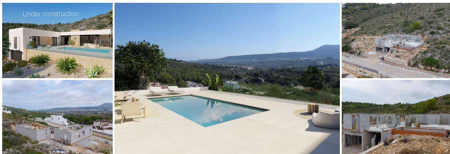
Modern new-build villa under construction for sale in Racó de Nadal, Benitachell
