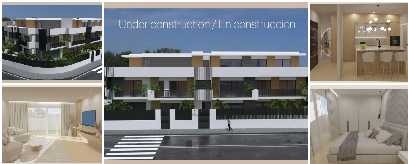
Apartment complex under construction in Jávea
