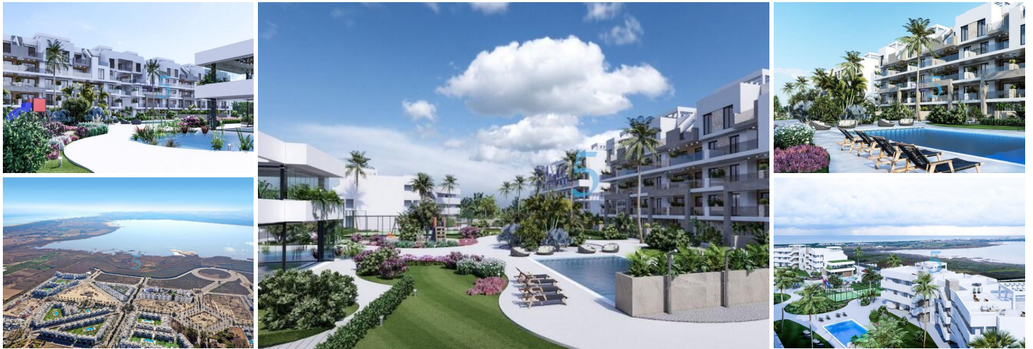
NEW BUILD RESIDENTIAL IN EL RASO, GUARDAMAR DEL SEGURA
