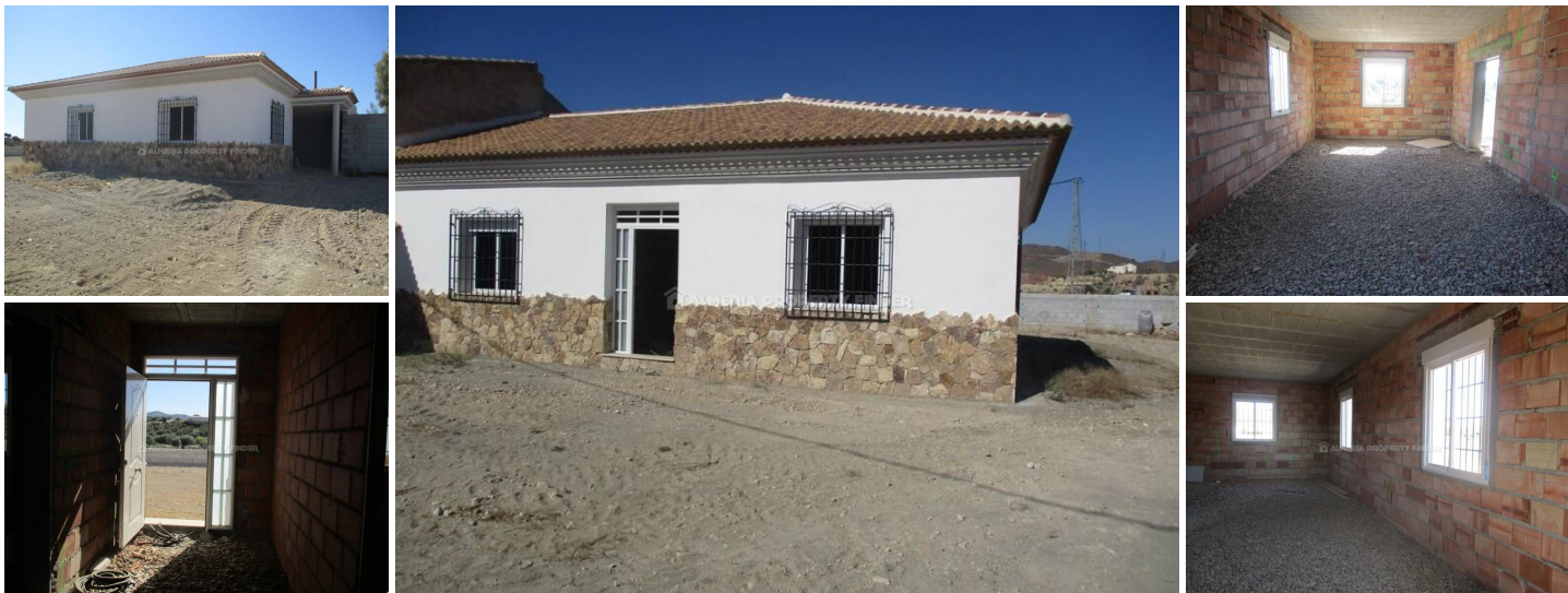
Villa Celeste - A villa in the Albox area. (Under Construction)
