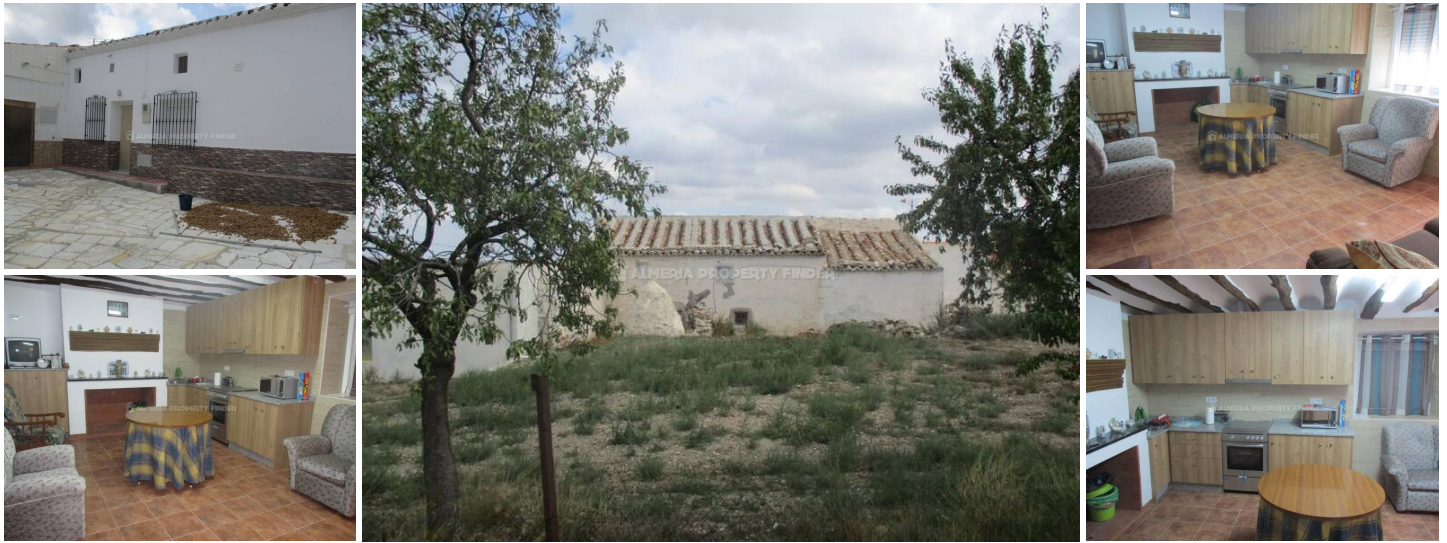
Cortijo Manzanas - A country house in the Velez Rubio area. (Partially Reformed)
