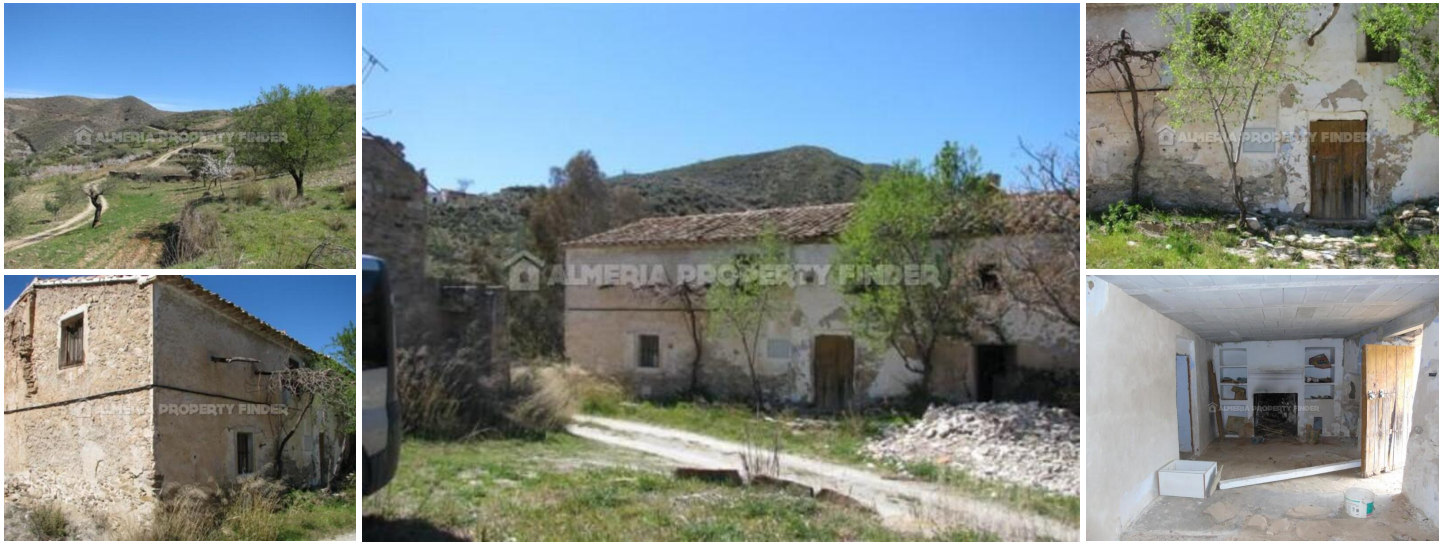
Ruina Rustica - A country house in the Lubrin area. (For Renovation)
