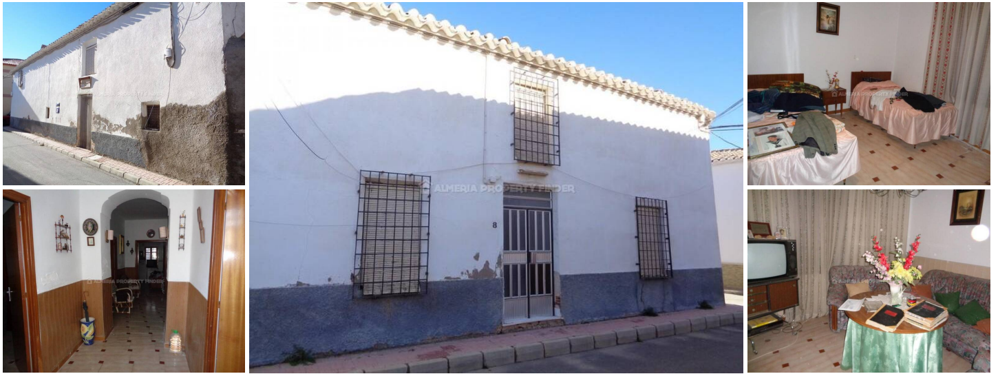
Casa Tania - A village house in the Albox area. (Habitable)
