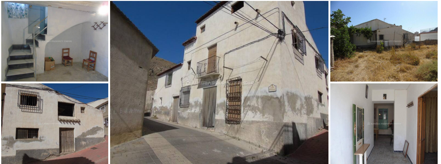
Casa Luciana - A town house in the Oria area. (Partially Reformed)
