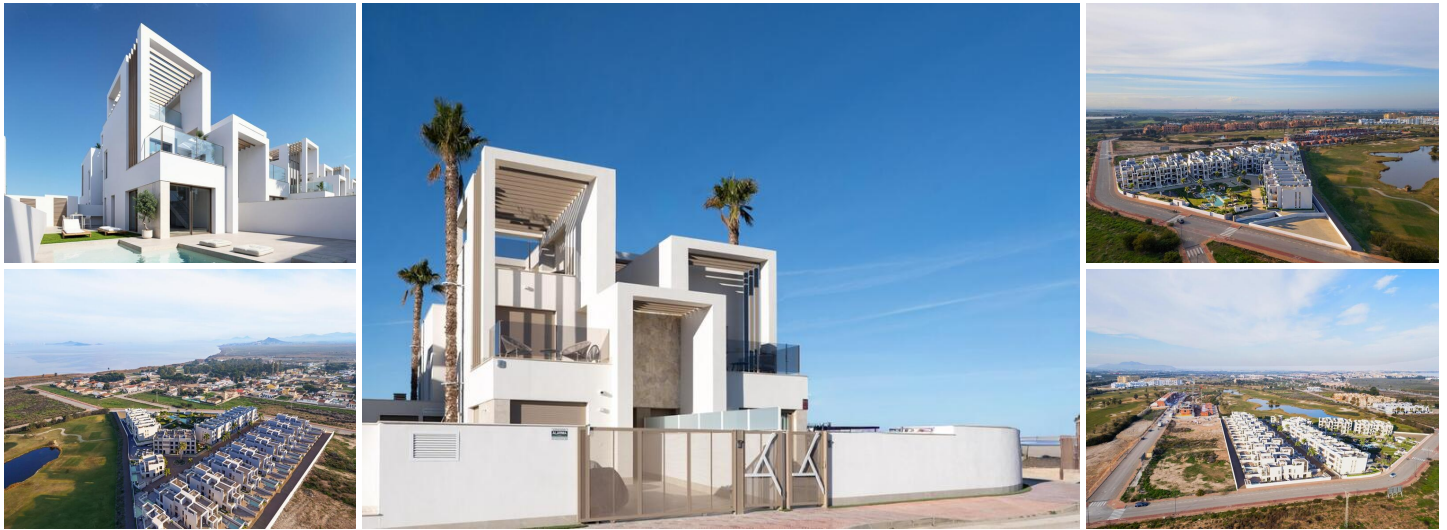
New Build Villas with Private Pool at Serena Golf-Los Alcazares
