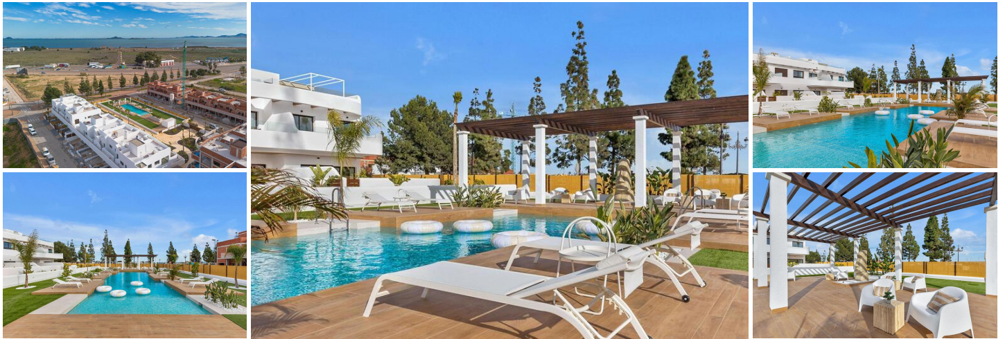
New Build Residential Complex Near Serena Golf and the Mar Menor in Los Alcazares
