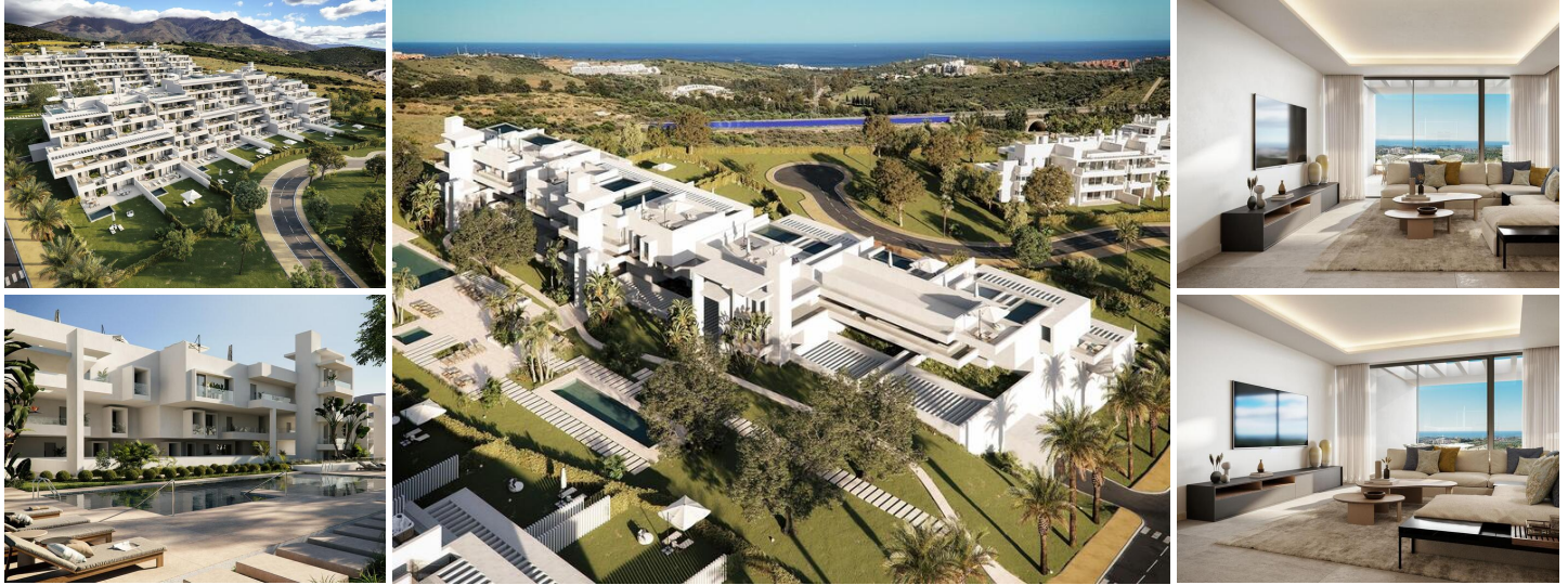
NEW BUILD RESIDENTIAL COMPLEX IN CASARES
