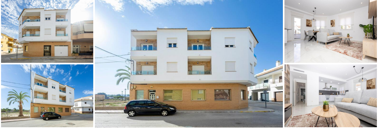
New Build Apartments in Jacarilla, Alicante
