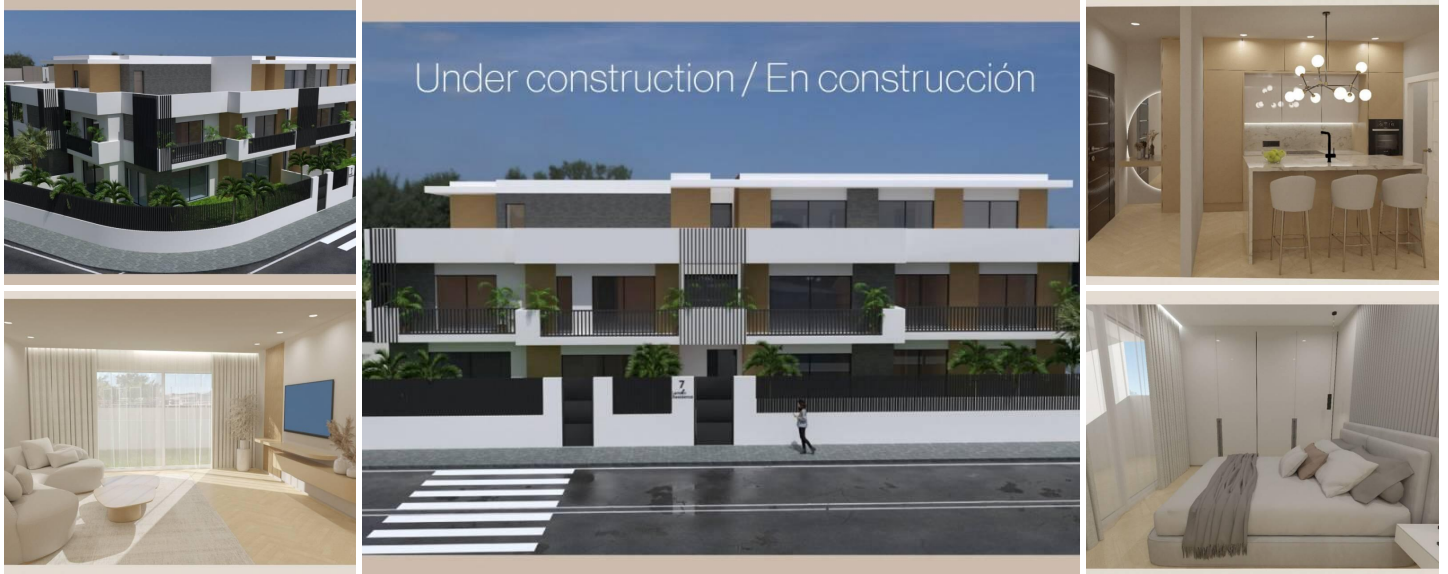
Apartment complex under construction in Jávea
