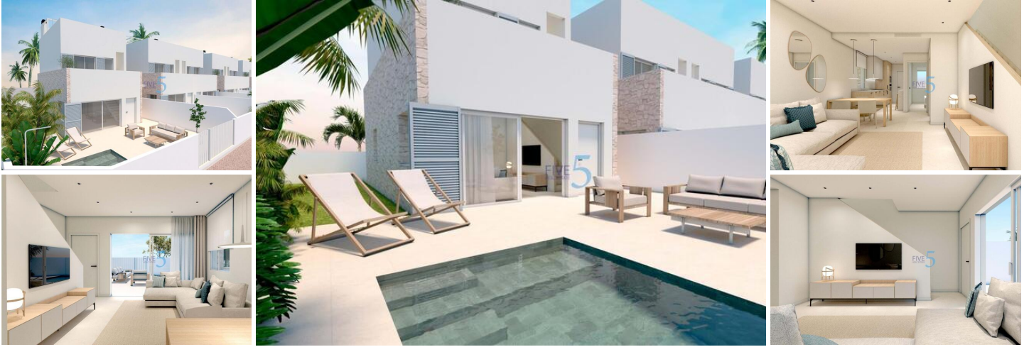
NEW BUILD VILLA IN TORRE DE LA HORADADA
