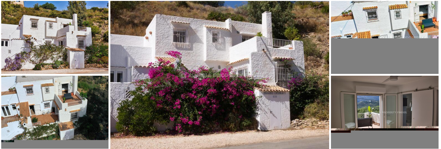
Town House Porter I - A town house in the Turre area. (Resale)
