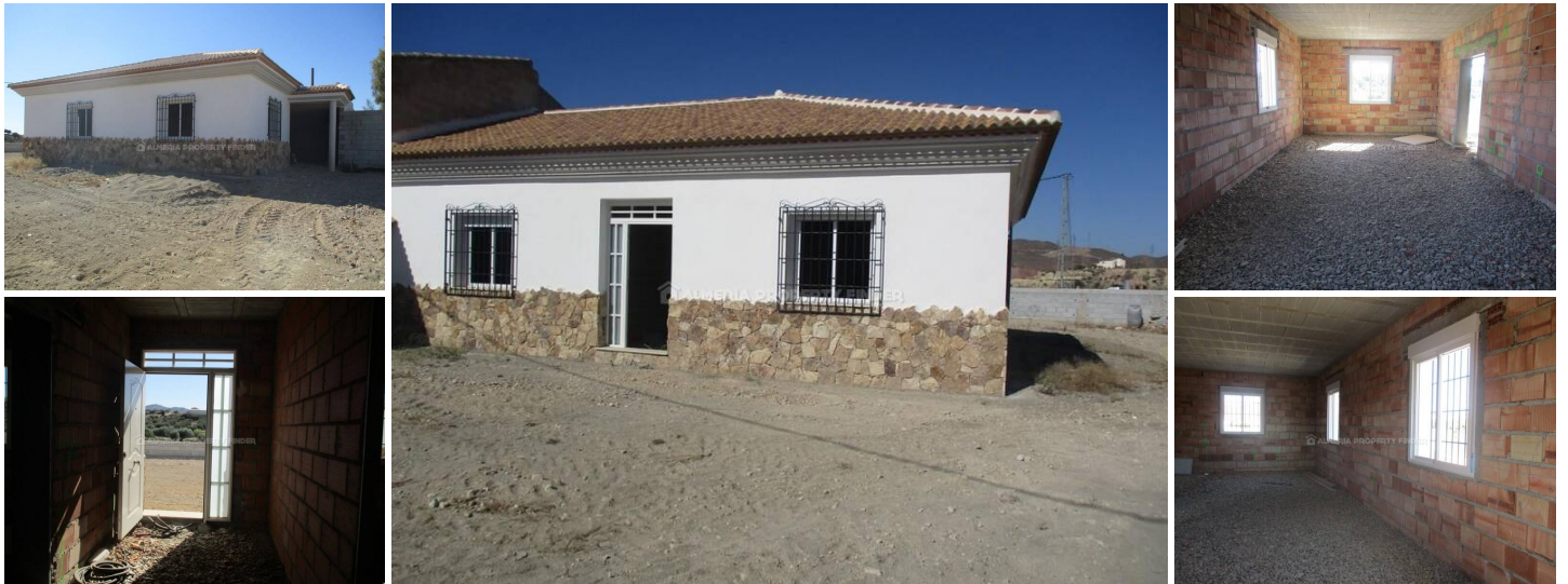
Villa Celeste - A villa in the Albox area. (Under Construction)
