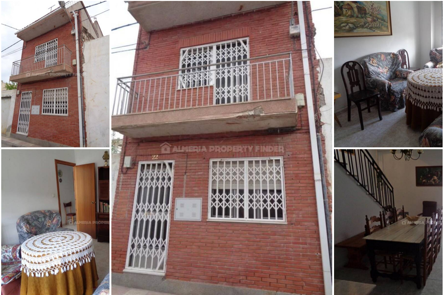
Casa Rubio - A town house in the Cantoria area. (Habitable)
