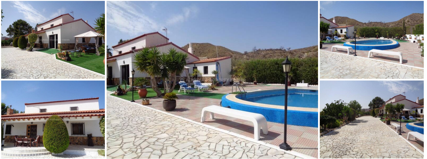
Casa Sanchez - A country house in the Arboleas area. (Renovated)
