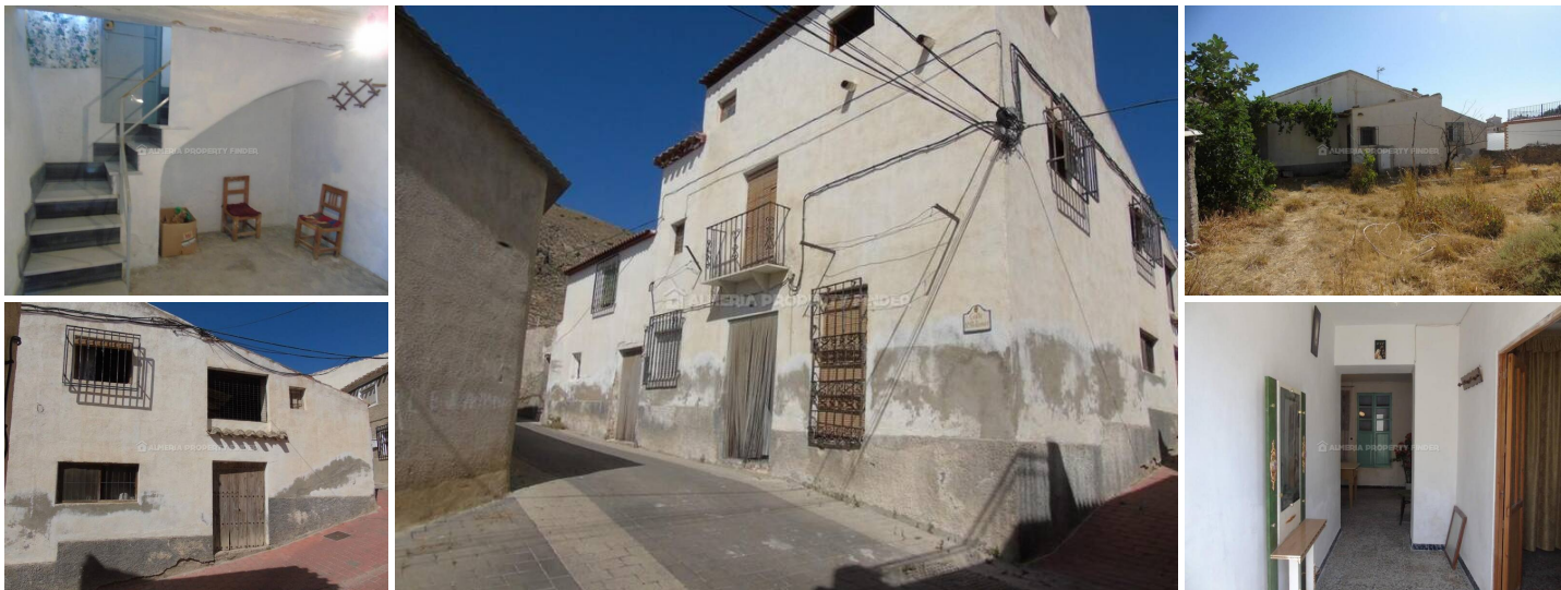
Casa Luciana - A town house in the Oria area. (Partially Reformed)
