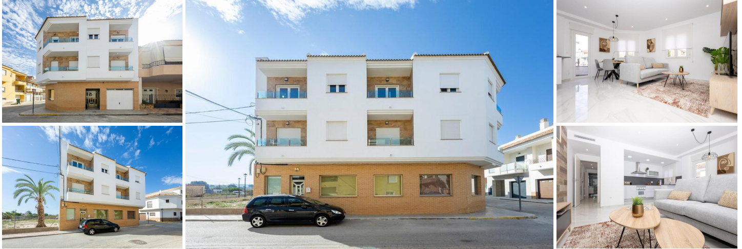
New Build Apartments in Jacarilla, Alicante
