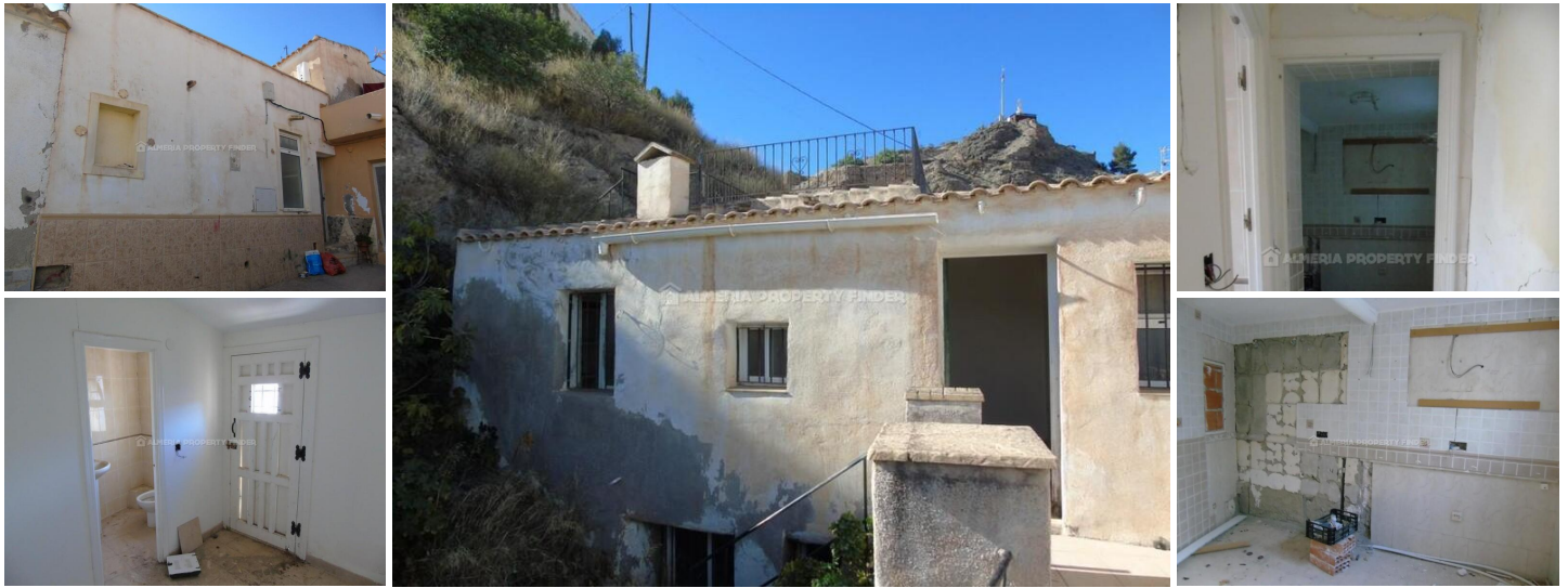
Casa Renata - A town house in the Purchena area. (For Renovation)
