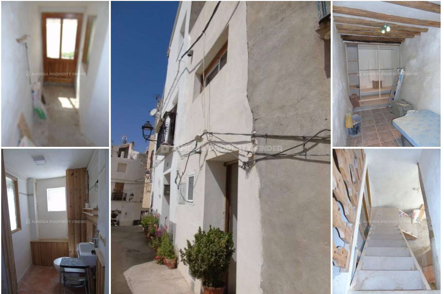
Casa Quesadas - A town house in the Seron area. (Partially Reformed)
