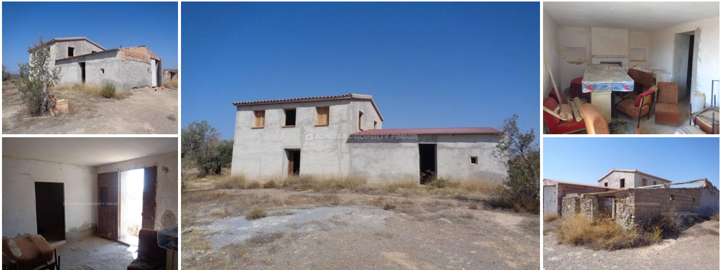
Cortijo Berbel - A country house in the Partalaoa area. (For Renovation)
