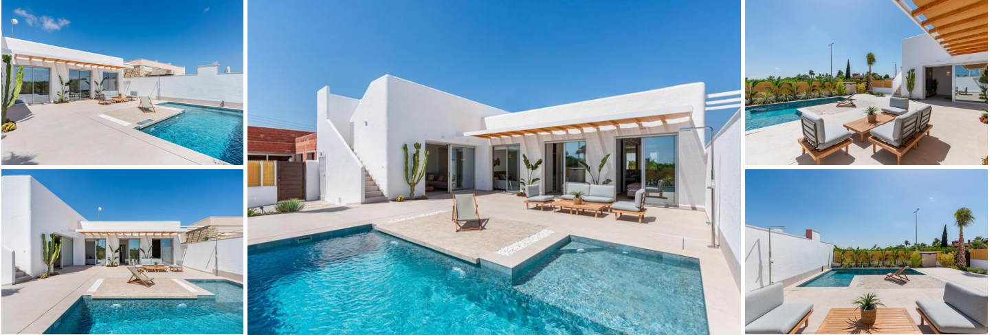
NEW BUILD VILLAS IN BENIJOFAR
