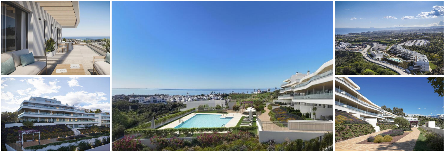
New Build Apartments with Sea Views next to Selwo Park, Estepona
