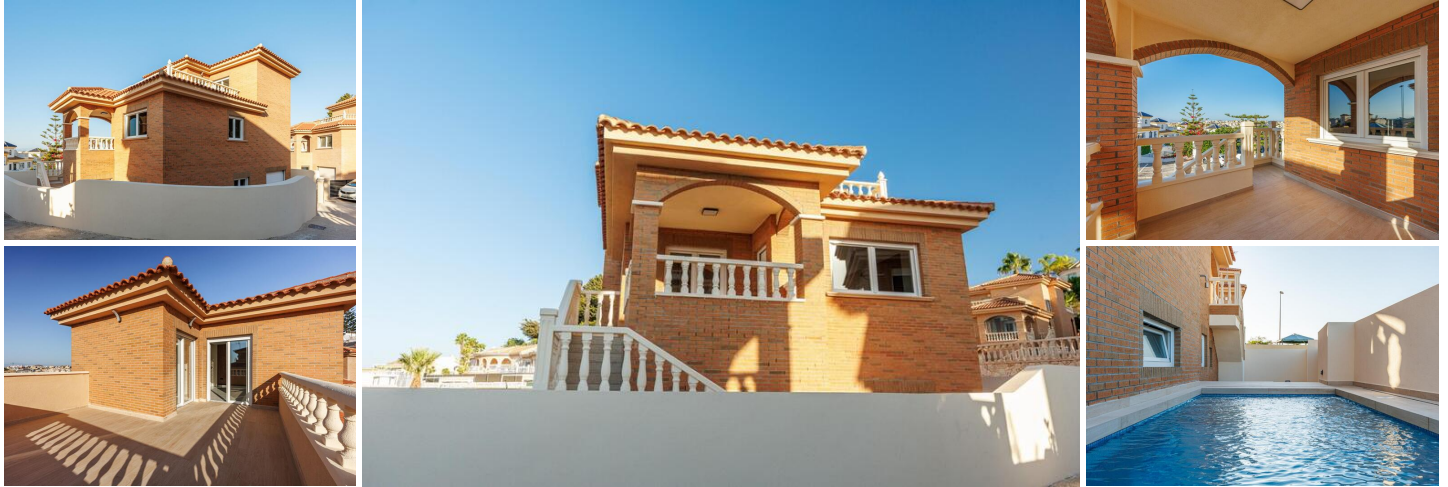
NEW BUILD VILLA IN ROJALES
