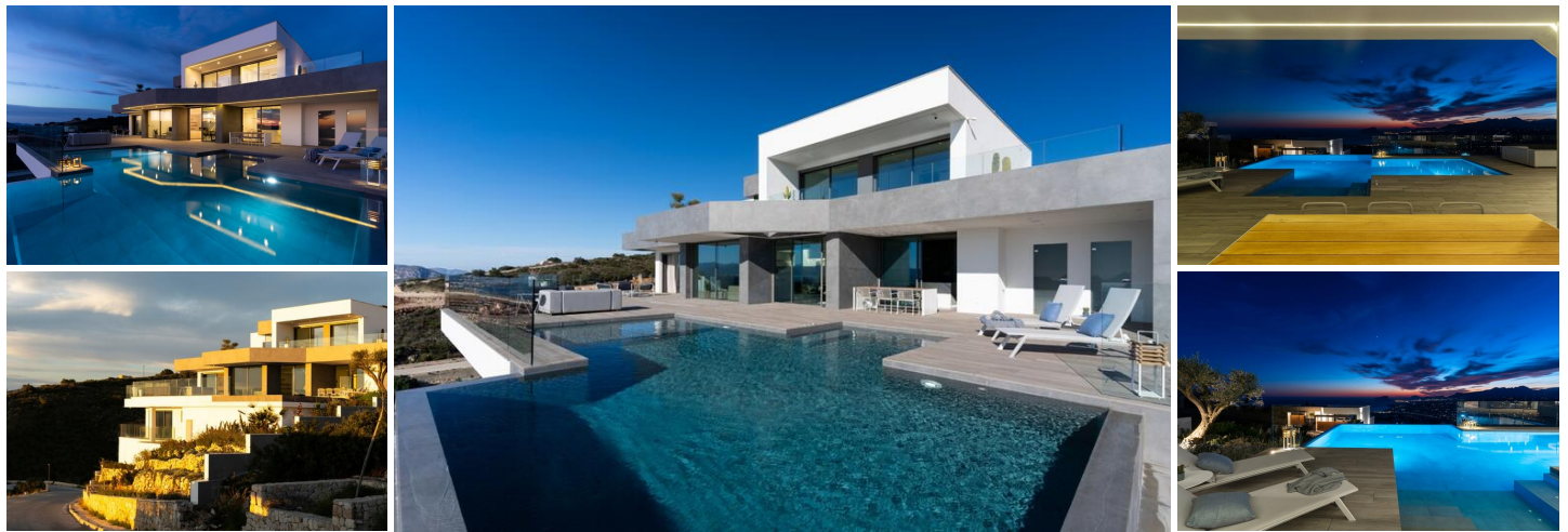
Villa Turnkey Luxury in Cumbre del Sol
