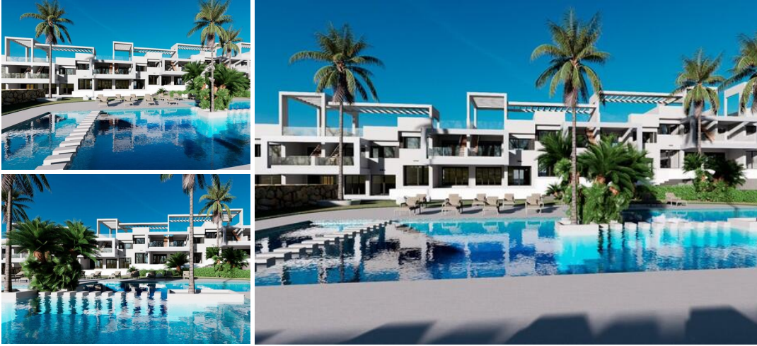
NEW BUILD RESIDENTIAL COMPLEX IN FINESTRAT
