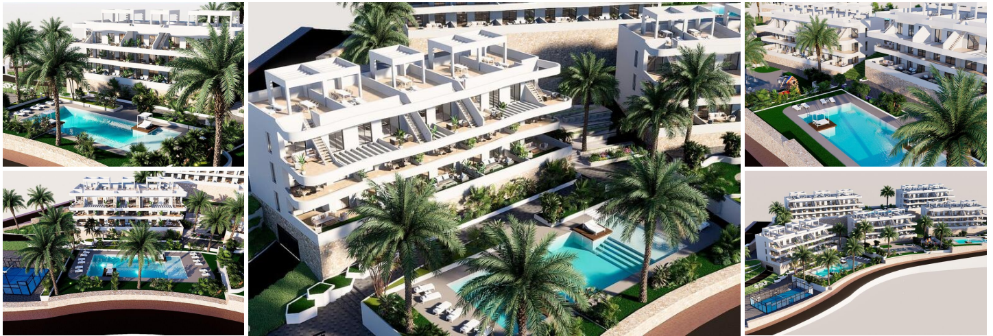
NEW BUILD RESIDENTIAL COMPLEX IN FINESTRAT
