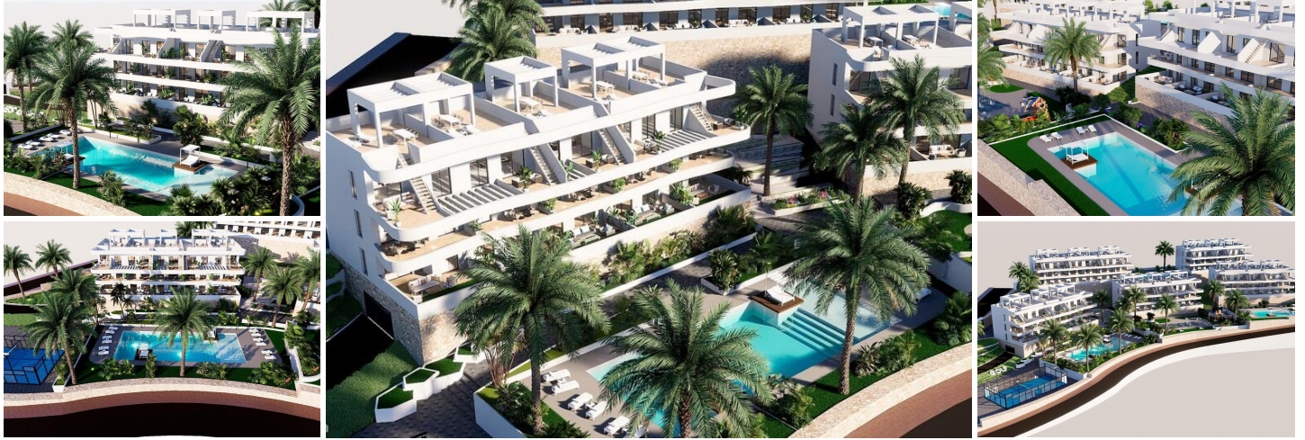
NEW BUILD RESIDENTIAL COMPLEX IN FINESTRAT
