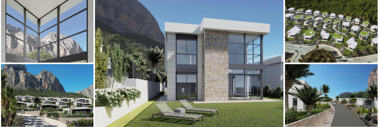
Neubau Villen in Polop, Alicante
