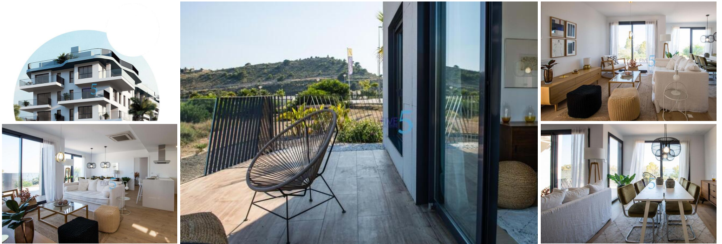
NEUBAU-KOMPLEX IN VILLAYOJOSA
