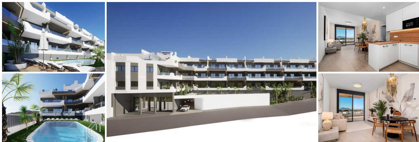
NEW BUILD BUILD RESIDENTIAL COMPLEX IN BENIJOFAR
