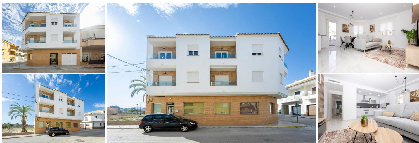
New Build Apartments in Jacarilla, Alicante
