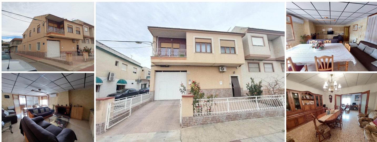
Semi detached 3 bedroom house in Desamparados Orihuela
