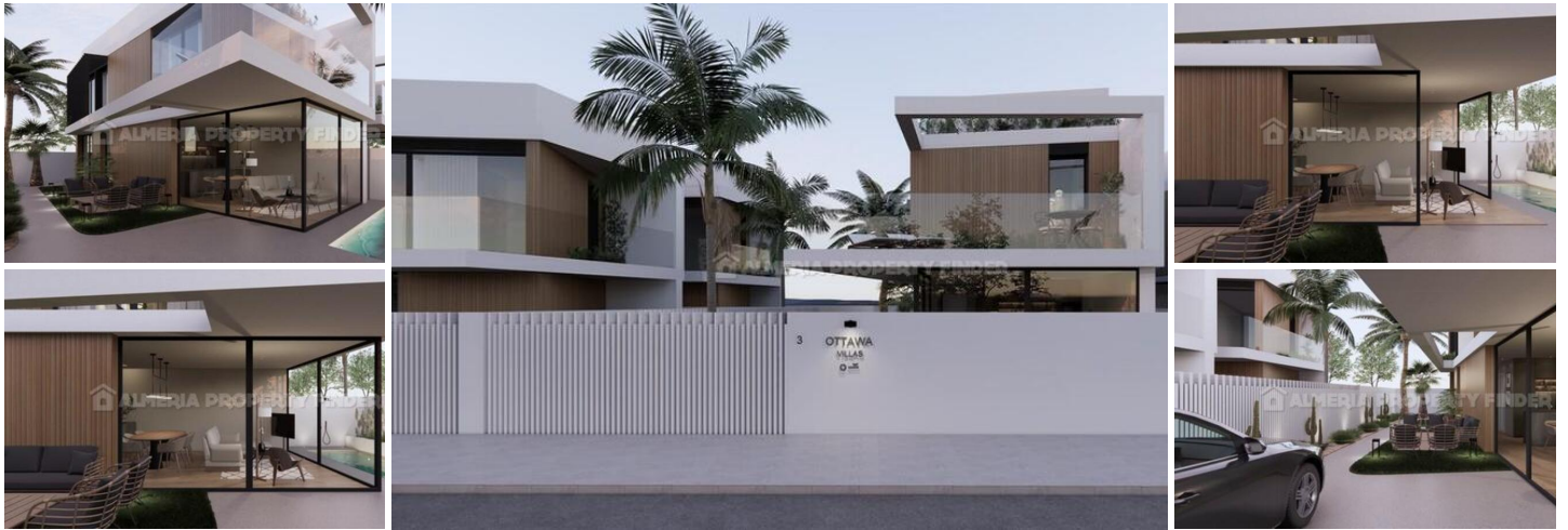
OTTAWA LUXURY VILLA 1A - A villa in the Torre de la Horadada area. (Under Construction)
