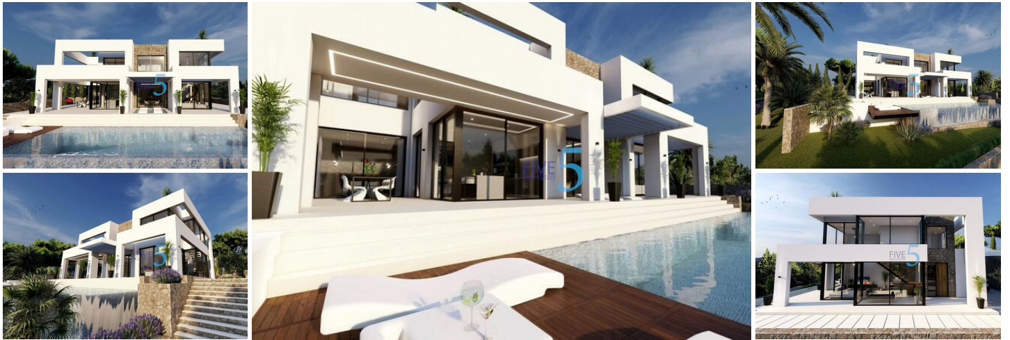
NEW BUILD VILLA IN BENNISA
