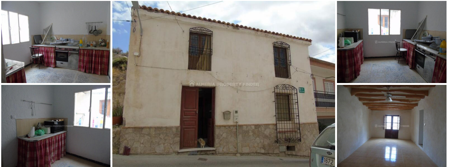
Casa Bodega - A town house in the Zurgena area. (Partially Reformed)
