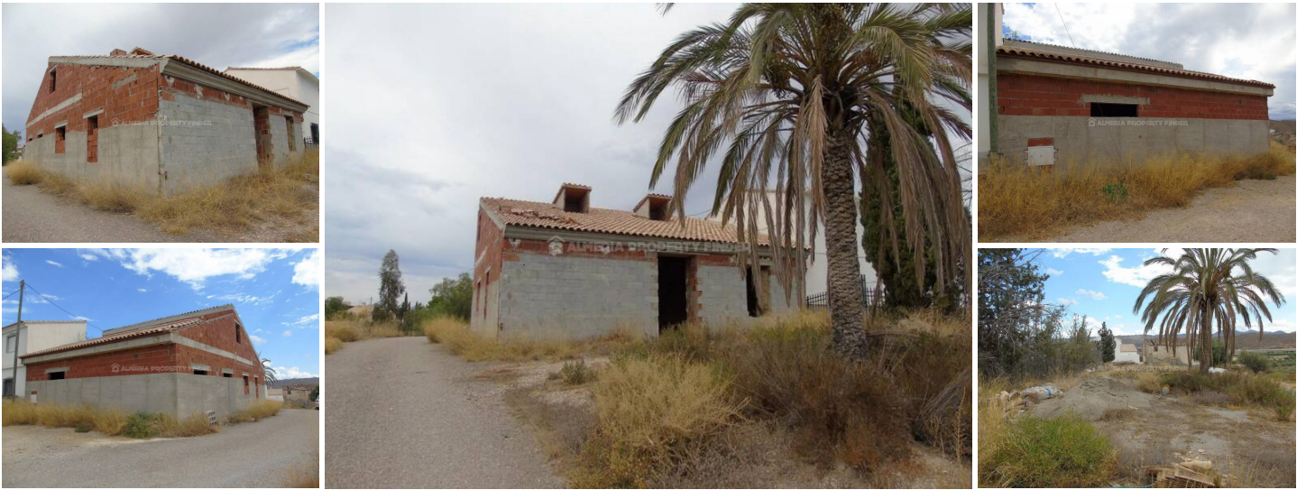
Casa Canico - A country house in the Albox area. (Under Construction)
